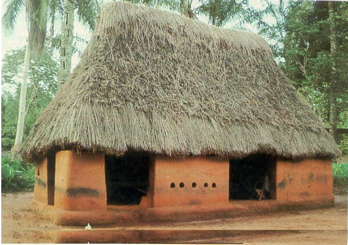
Photograph 1. Igbo Architecture as a Symbolic System adapted from Aniakor, (1989: 52). "The State of Igbo Architectural Studies". In Journal of Igbo life and Culture Uwa ndi Igbo Vol. 2. Nsukka, Okiki Arts Centre. The above picture is a typical Obi/Obu house in various Igbo communities. Every Obi/Obu is strategically positioned on every compound in such a way that the mgboezi faces it directly. It is this structure that is ritually cleansed and taken over by the first son through the Ikpocha Obi ceremony. The researcher came across this particular photo in a book Igbo Architecture as a Symbolic System by written by Aniakor (1989: 52) at the University of Nigeria Library.
