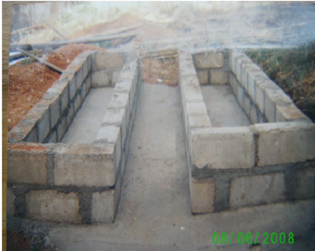
Figure 5. Construction of an anaerobic digester.
