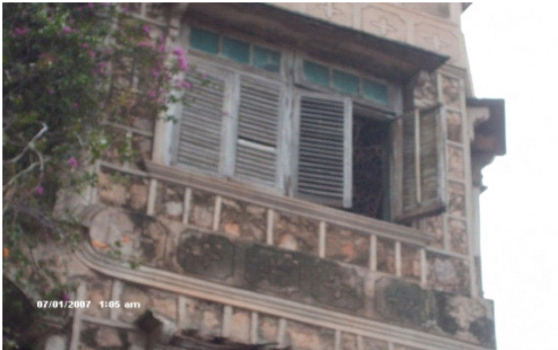
Figure 5. The stone rubble walls of Sussan Wenger's Building, Osogbo, Nigeria.
