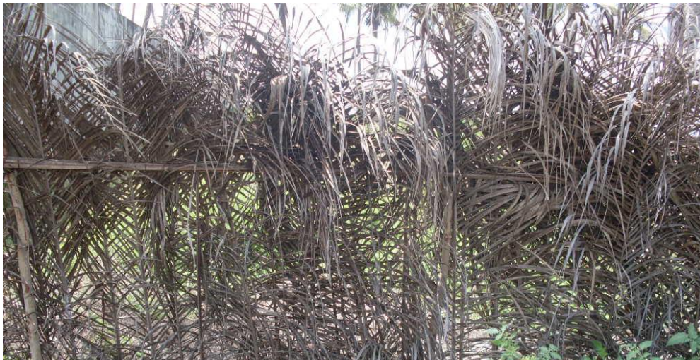
Figure 5. Method of palisade set up to abate the effect of tidal breeze
