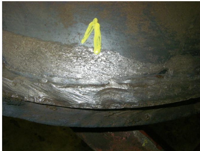
Figure 9. Zone of crack propagation, point 1, failure initiation and crack propagation.
