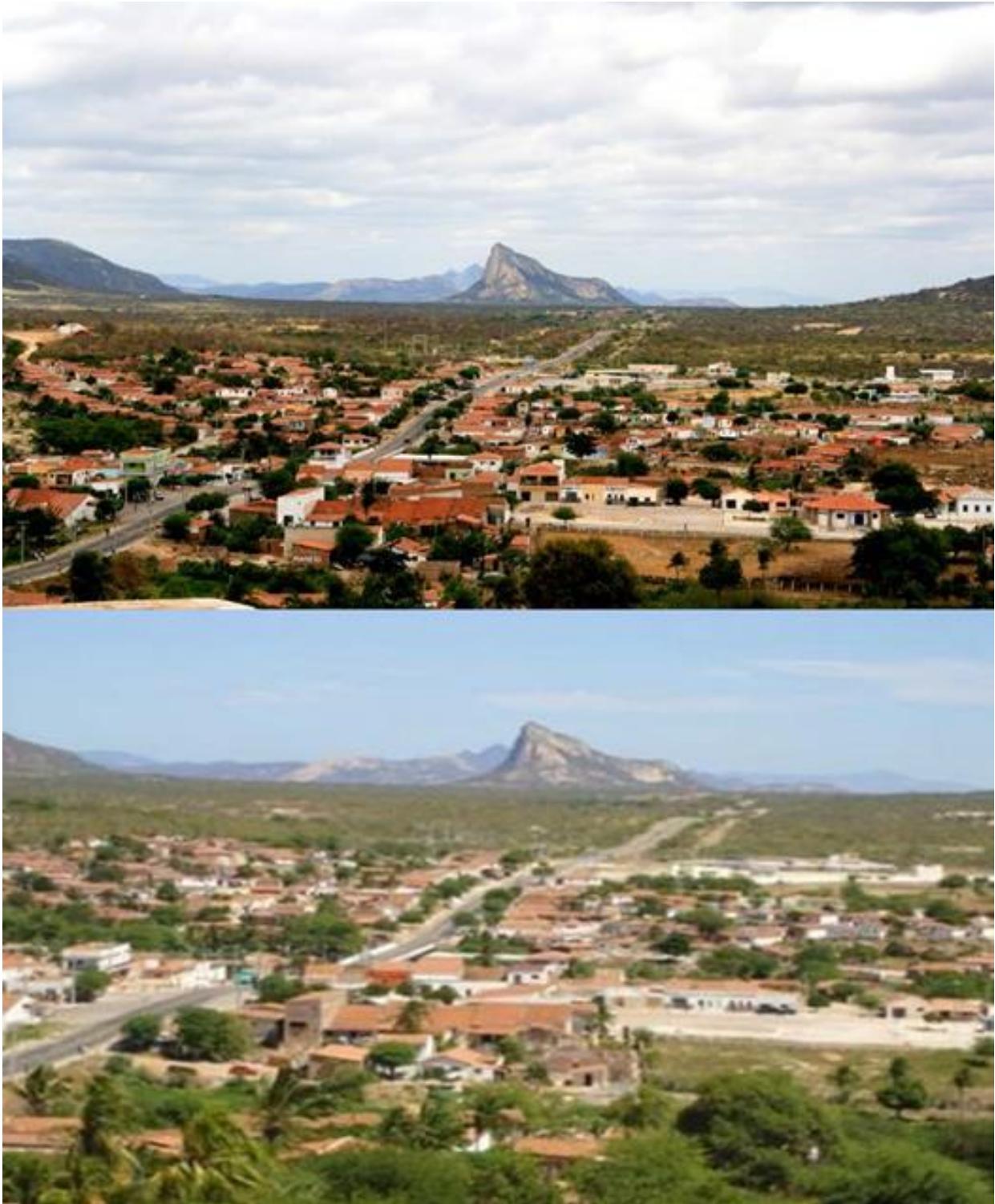
Figure 2. Hospital and Maternity Sinhá Carneiro located in the city of Santa Luzia, Paraíba (Source: Mayara, T. Santos).
