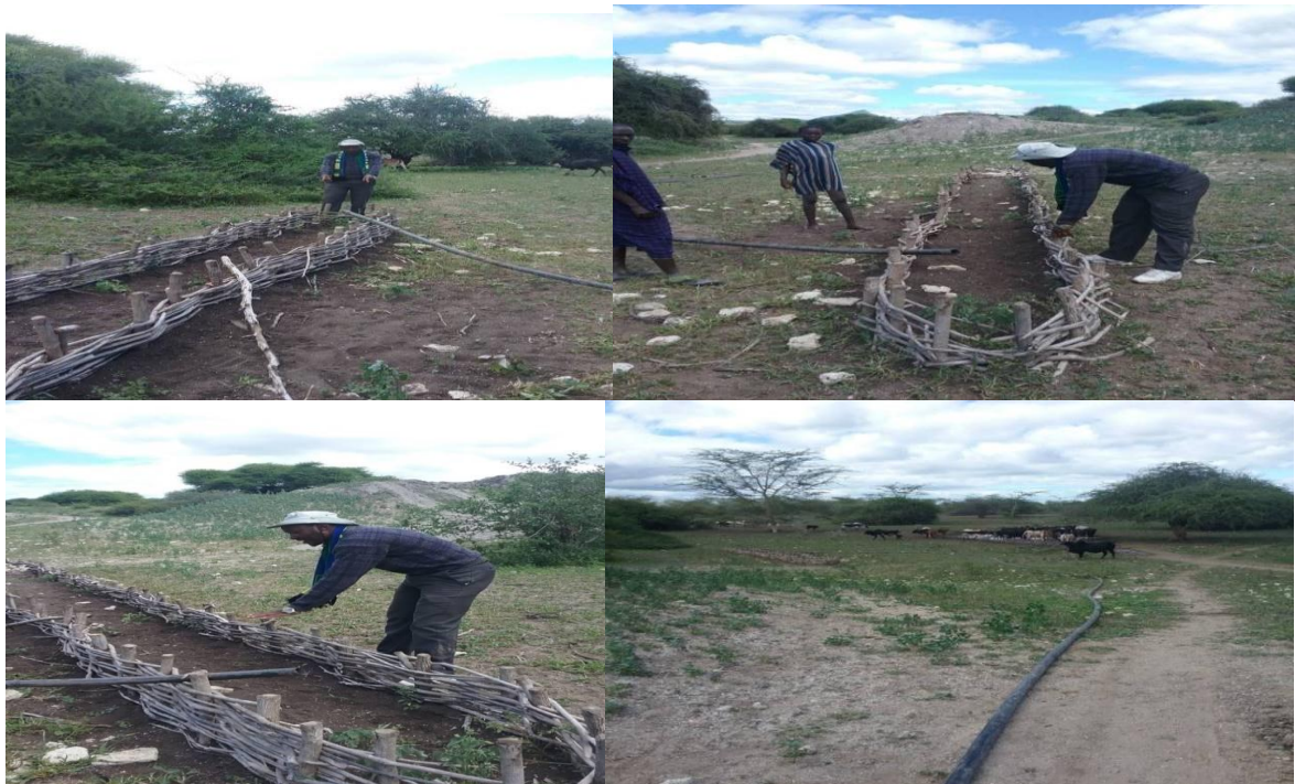
Figure 14a. The old Water Reservoir/Mboutu at Makame, Ndedo and Saunyi villages.
