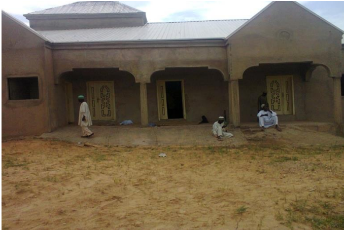
Plate X: Front view of the uncompleted site Museum.
