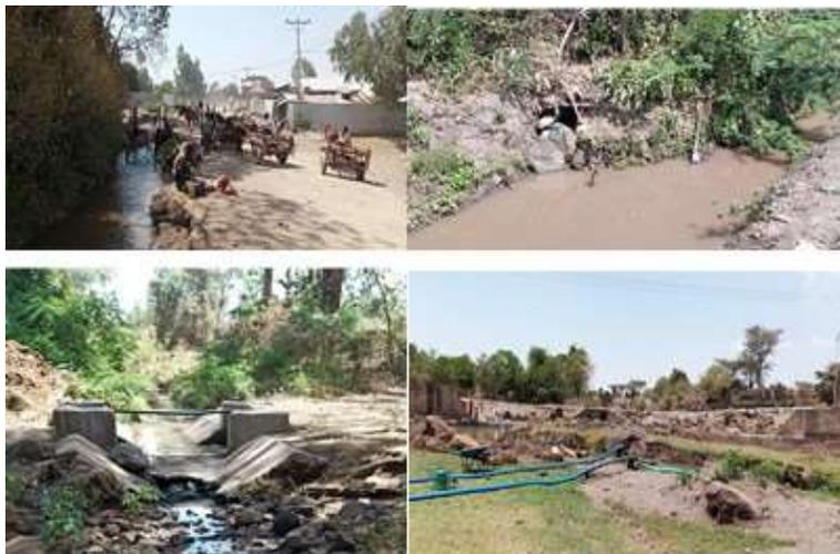
**Figure 5.** Breached structures, stone-regulated offtake, fully silted diversion weirs, and multi-use supply canal at Ketar and Arata Irrigation schemes. Source: Pictures taken in March 2021 as a part of data collection by the researcher.
