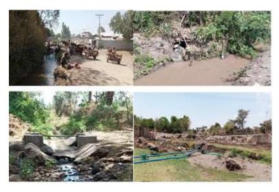
**Figure 5.** Breached structures, stone-regulated offtake, fully silted diversion weirs, and multi-use supply canal at Ketar and Arata Irrigation schemes. Source: Pictures taken in March 2021 as a part of data collection by the researcher.
