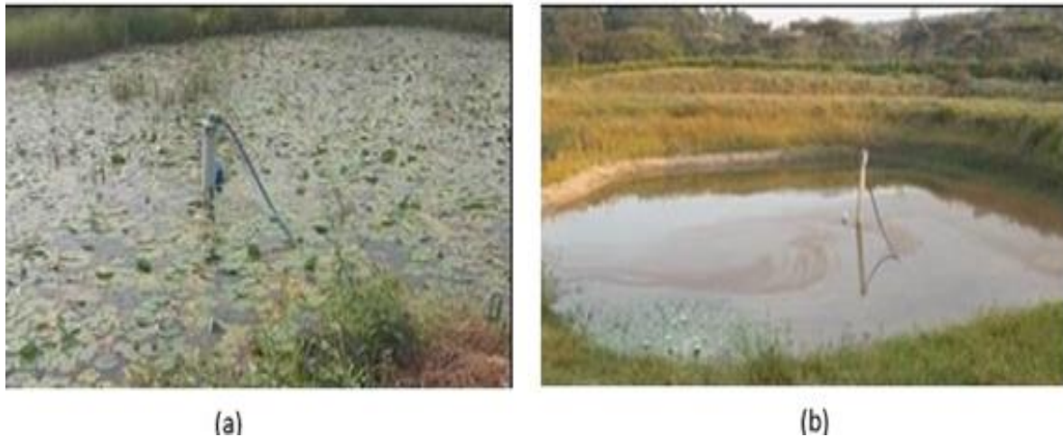
Figure 4. Previously installed submersible solar pump in the valley tank. Source: Submersible pump installation in a reservoir for Mawokota Farmers' Association (Mpigi district)
