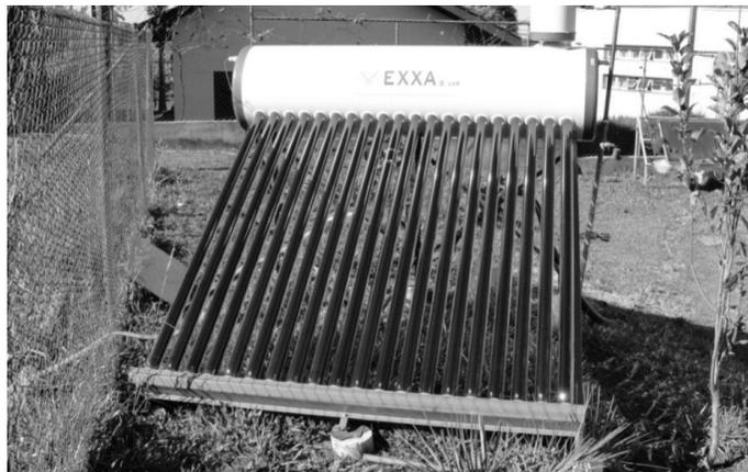
Figure 1. Solar collector with vacuum tubes type all-glass.
