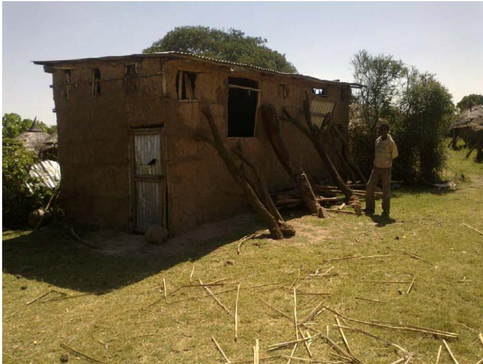
**Plate 2.** Termite infested houses supported by poles.
