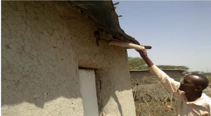
**Plate 1.** A roof supporting timber completely cut by termites.
