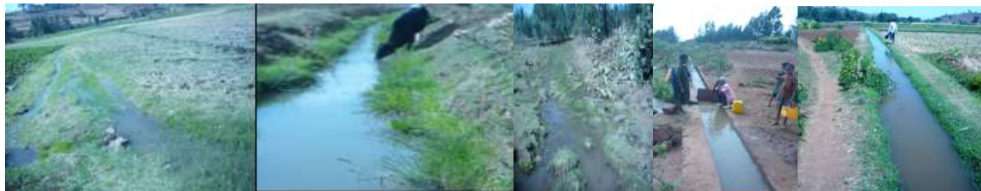
Figure 2. Overflowing of unlined canals and livestock interference at Selamko (left 3) and lined and unlined main canals at Shina-Hamusit (right 2) irrigation schemes.
