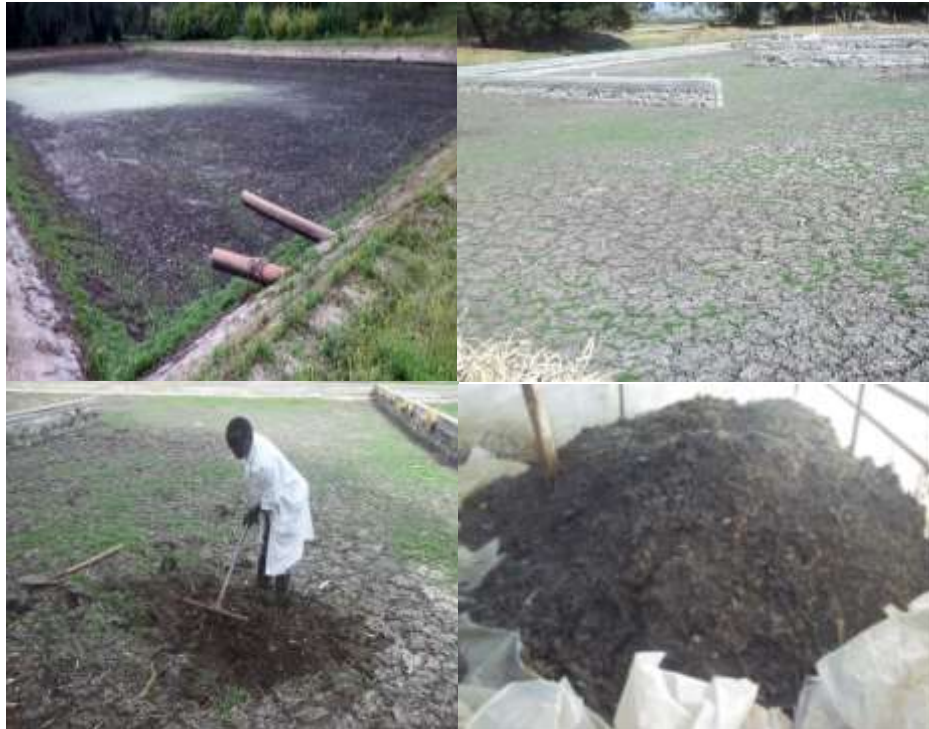
Plate 1. Harvesting of biosolids in the sixth (semi solid) and seventh (dry) lagoons.
