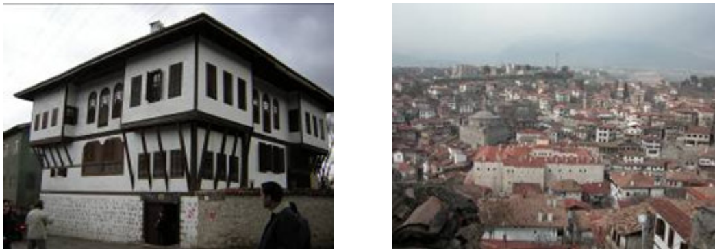
Figure 6. Traditional houses in Safranbolu, built in the early 1900s.
