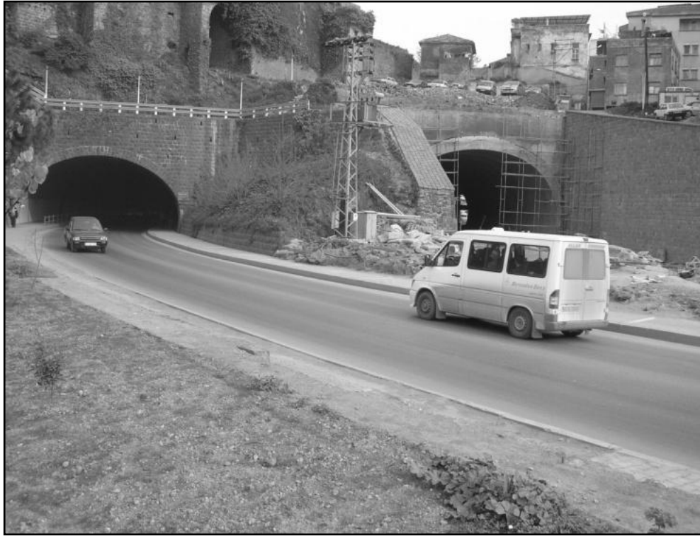
Figure 5. Trabzon city bypass tunnels.
