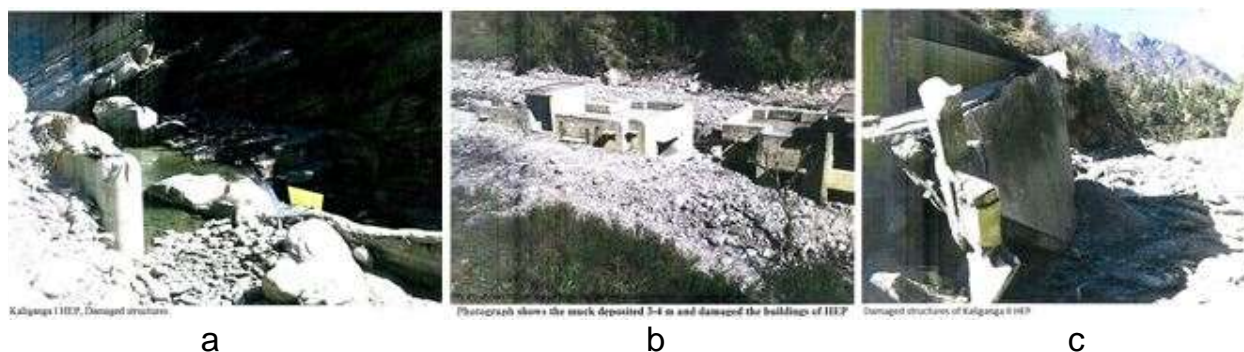
Figure 29. (a) Kali Ganga I HEP (4 MW, Rudraprayag District) ( https://sandrp.wordpress.com/2014/06/16/uttarakhand-flood-disaster-of-june-2013-lest-we-forget-the-experience-and-its-lessons/ ); (b) Kali Ganga II HEP (6 MW, Rudraprayag district, Mandakini Basin), muck-deposited 3-4 m that damaged the building of HEP ( https://sandrp.wordpress.com/2014/06/16/uttarakhand-flood-disaster-of-june-2013-lest-we-forget-the-experience-and-its-lessons/ ); (c) The damaged structures of Kali Ganga II HEP.
