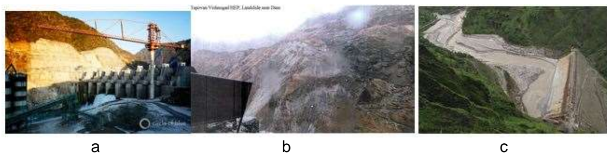
Figure 27. (a) Srinagar Hydroelectric Project on Alaknanda river, India Srinagar HEP - Source: http://www.circleofblue.org/waternews/2014/world/uttarakhands-furious-himalayan-flood-bury-indias-hydropower-program/ (left inset); (b) Land slide near the dam of Tapovan Vishnugad HEP ( https://sandrp.wordpress.com/2014/06/16/uttarakhand-flood-disaster-of-june-2013-lest-we-forget-the-experience-and-its-lessons/ ) (middle inset); (c) The Dhauliganga hydropower dam after being flushed off of bed-load sediment following 2013 Flood ( http://sandrp.wordpress.com/2013/09/27/uttarakhand-floods-of-june-2013-curtain-raiser-on-the-events-at-nhpcs-280-mw-dhauliganga-hep/ ).
