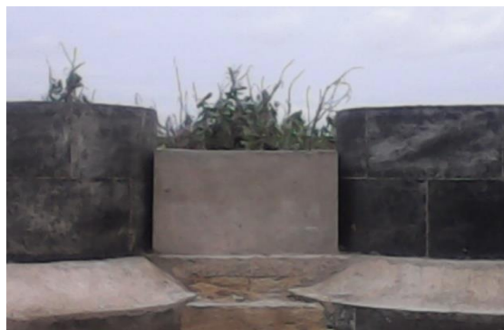
Figure 1. 2 Digesters of PUXIN model.
