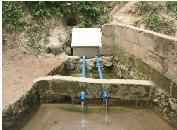
Figure 1. Awedele Spring showing concrete protection.
