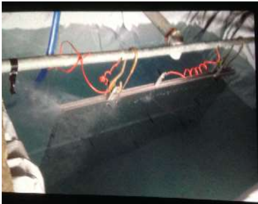
Figure 2. Electro-defluoridation system installed at Berta-Sembi communities in the Rift Valley of Ethiopia (Photo by Teshome L. Yami).
