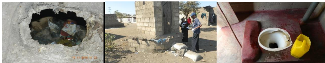
Figure 8. Example of latrine construction and interfaces that discourage direct latrine usage by young children from Kanyama study area.
