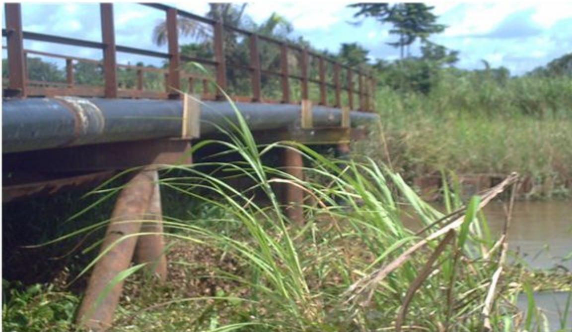
Plate 1. On-going metal construction work at sampling station 6.
