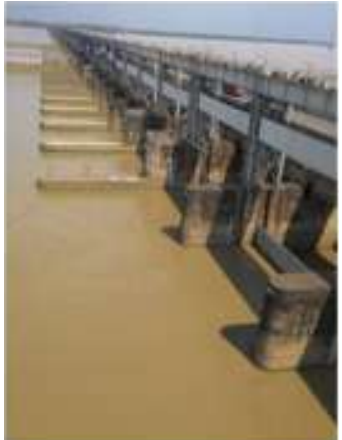
Figure 12. The 2,245 m long Farakka Barrage with 109 gates, 18.30 span, and 76,500 cumecs discharge capacity upon the Ganges (courtesy of SANDRP – South Asia Network on Dams, Rivers and People) Thakkar (2017).
