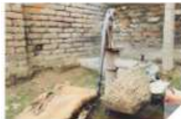
Figure 48. Deserted hand tubewells either fail to extract groundwater or yield arsenic-contaminated water. Source: Photo credit: Samad, 2003, personal communication)
