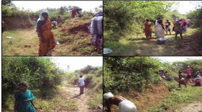
Figure 3. Execution of desilting of channel work in the Avalur Village.
