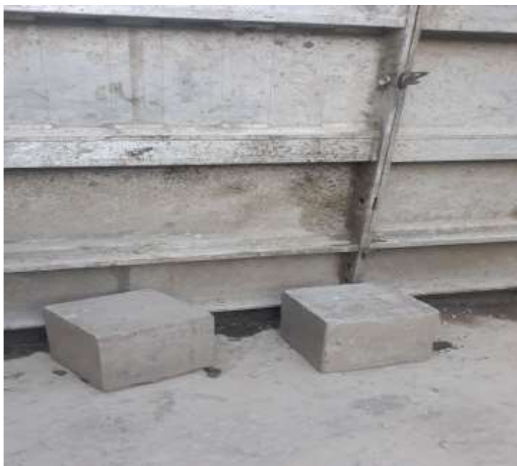
Photo 3. Samples curing along with permanent concrete structures.
