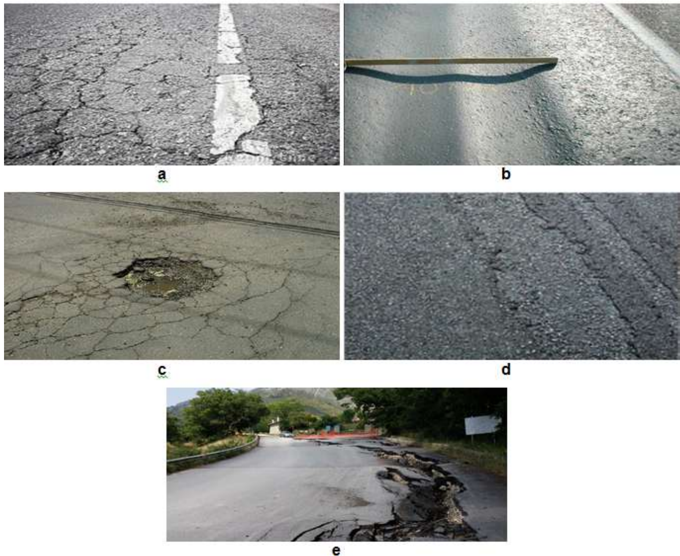
Figure 1. (a) Alligator cracking; (b) Rutting at wheel path; (c) Potholes; (d) Ravelling; (e) Block cracking.
