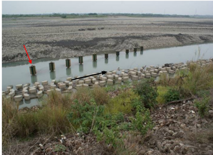
Picture 1. Study reach, Laonong river, photo facing left bank. Black arrow denotes flow direction; red arrow indicates position for groin-head.
