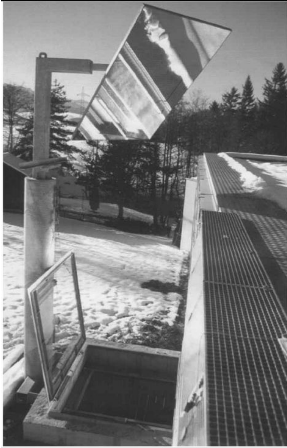
Figure 6. Sun lighting system redirection mirror (Carter, 2004:224).
