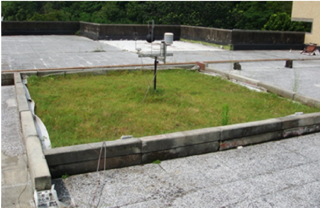
Figure 1. A five meter square lawn planted area with 13 cm substrates underneath were created at the centre of a building's rooftop.
