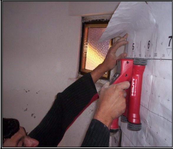
Figure 2. Scanning with a ferroskan device.
