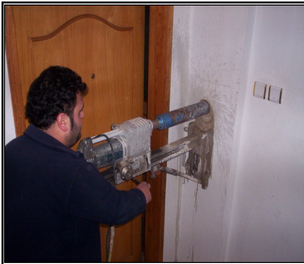
Figure 3. Coring from concrete wall with a portable water-cooled drilling machine.
