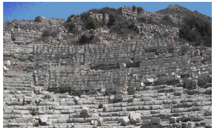
Figure 17. Sample of stones being marked and that are belonging to east part of Knidos Antique Theater.
