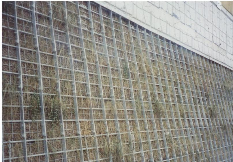
Photo 2. Slit wall constructed in in-situ test site.
