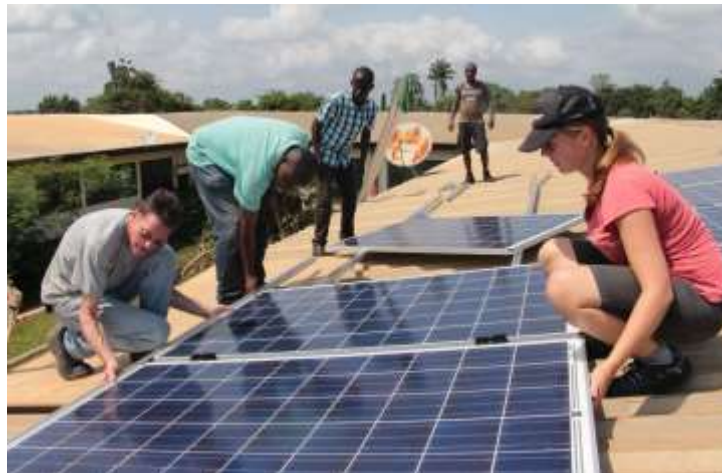
Figure 6. Installation of a photovoltaics hybrid system in Ghana (source: CIRE/TH Cologne)
