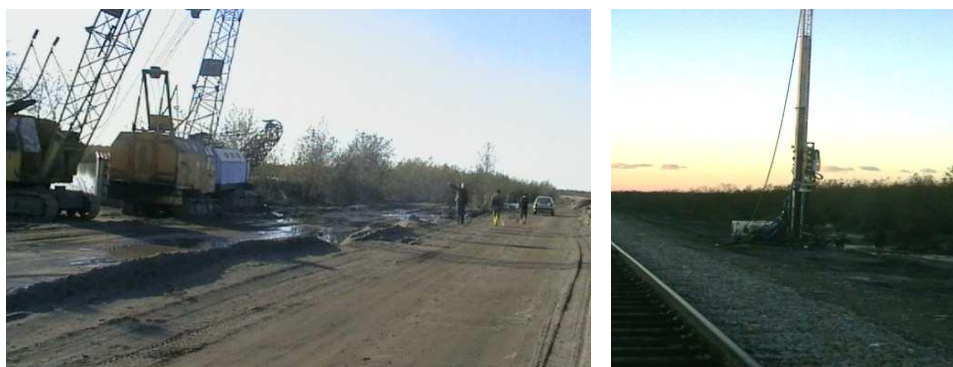
a. Stone column practice
