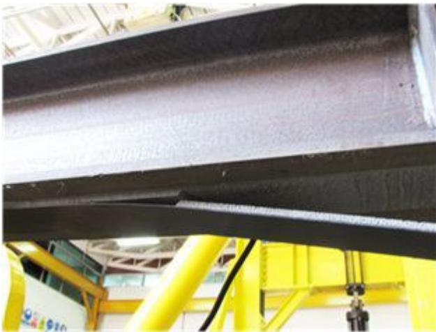
Figure 6. Below load debonding (BLD).
