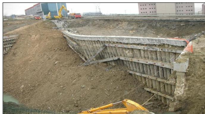
**Figure 12.** Collapsed Bored Piles
