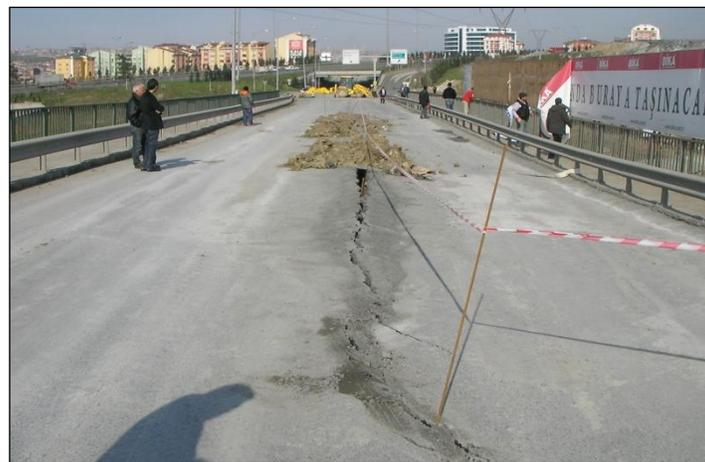
**Figure 8.** Expansions of the Cracks on the Road Embankment
