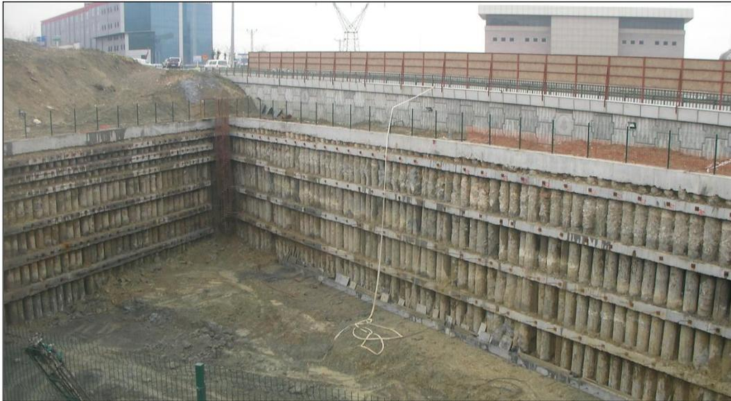
**Figure 1.** Non-deformed Condition of the Excavation Site
