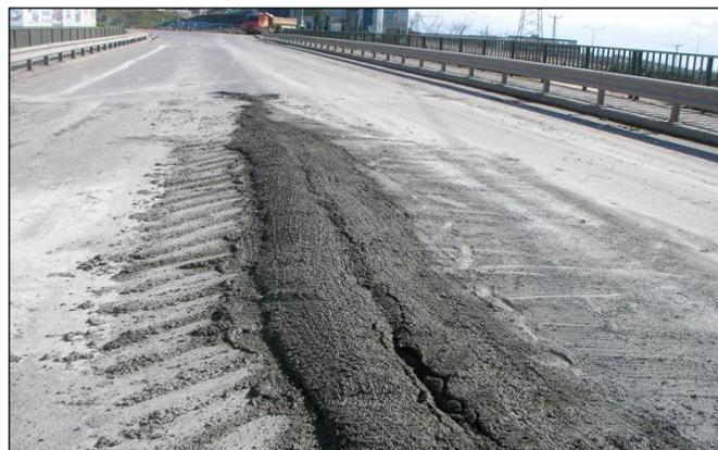
**Figure 9.** Filling of the Cracks with Concrete
