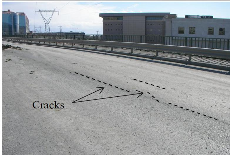
**Figure 7.** Deformations Occurred on the Road Embankment
