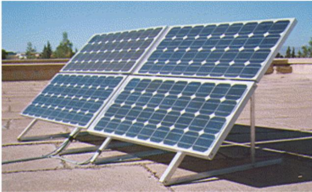
**Figure 15.** Photovoltaic panels SP75 (300 Wpeaks) installed at the laboratory.
