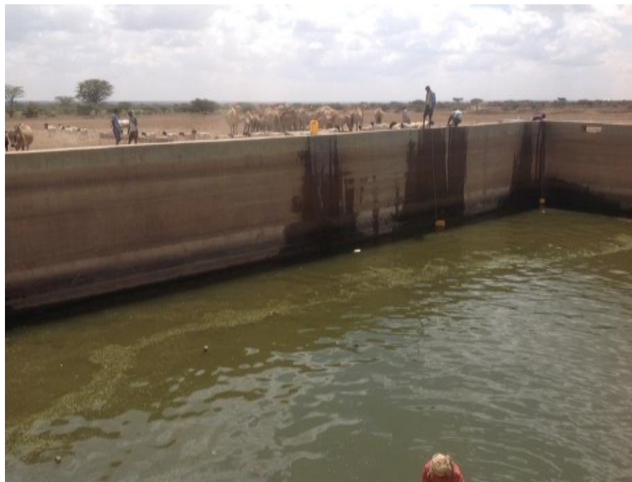
Photo 2. Public Birkas constructed for water collection in Chinkeda village. Source: Field Data (2015)
