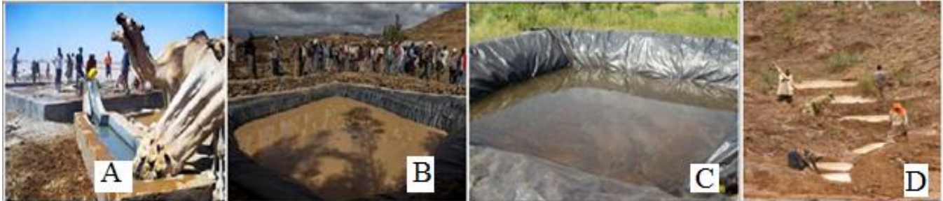
Figure 3. Water harvesting ponds using Geomembrane and micro basins in Ethio-Somali Region (A) and Amhara region (B-D) Ethiopia, respectively (www.gcca.eu/2014).
