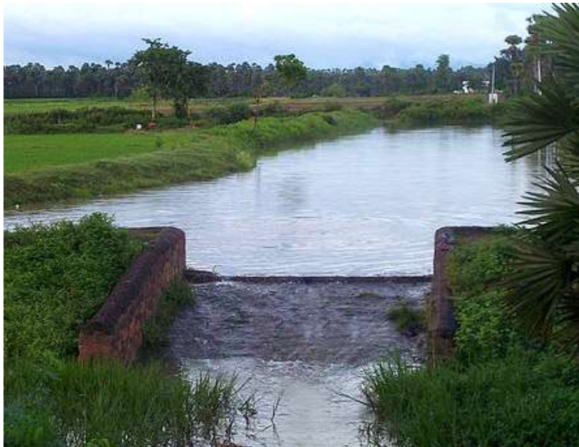
Figure 3. Another scene of Indian irrigation system. Tank (a reservoir of any specific size) irrigation in India( http://www.indianetzone.com/45/tank_irrigation_india.htm ).
