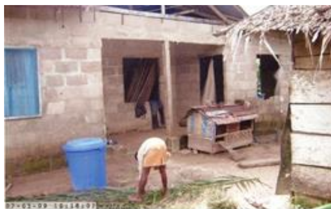
Figure 12. 4-bedroom bungalow being built by Madam Mercy at Obiota village.
