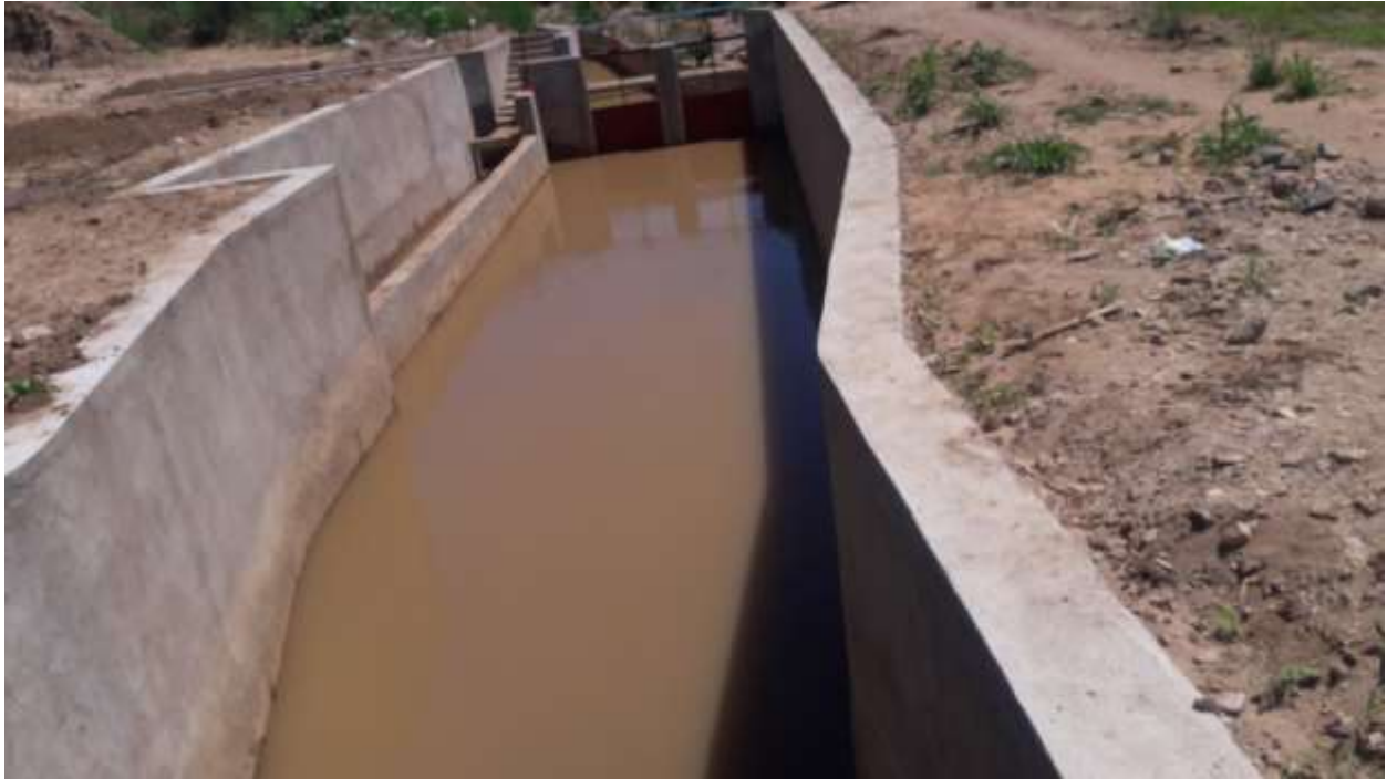
Figure 6. Magozi reconstructed water intake.
