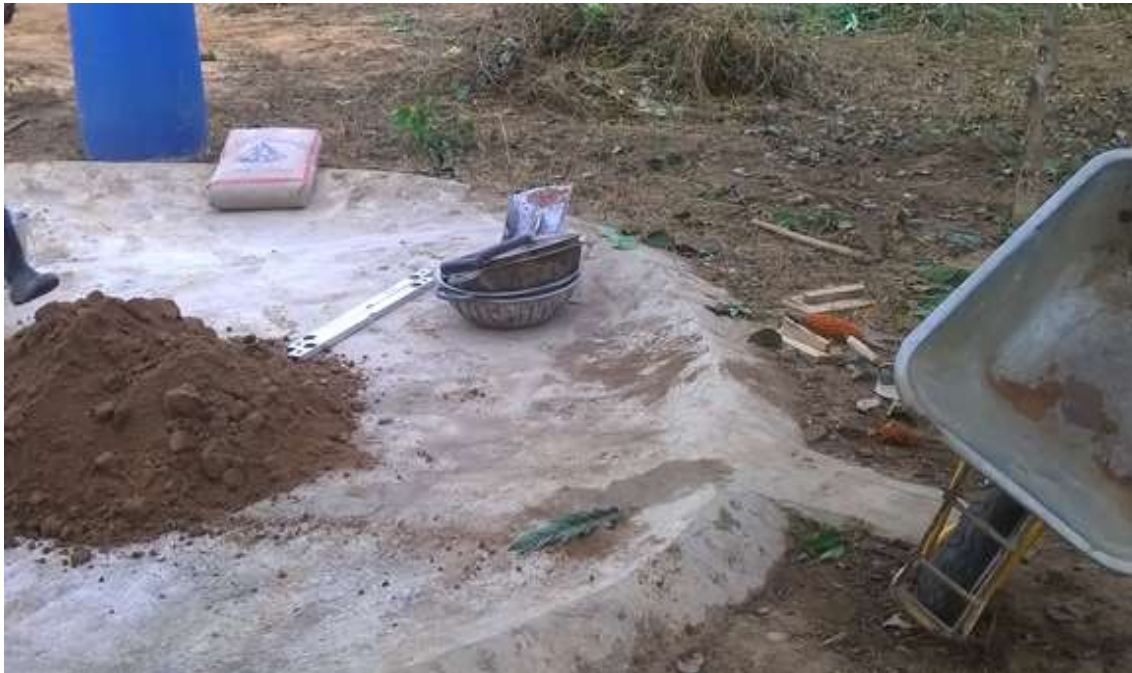
Figure 6. Some tools used by artisans on site. Source: Fieldwork (2016).
