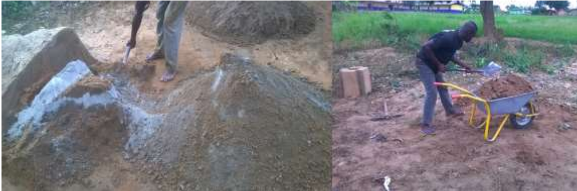
Figure 5. Eyeball batching as against volume batching using wheelbarrow by artisans on site. Source: Fieldwork (2016).
