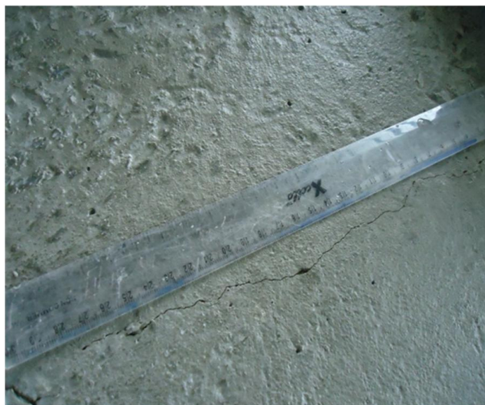
Figure 1. Shrinkage crack of Mix 1.
