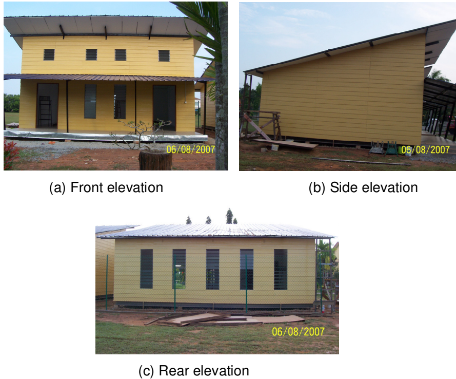
Figure 7. Plan and elevations of the school cabin module roofed with PSSDB roof in the present work.
