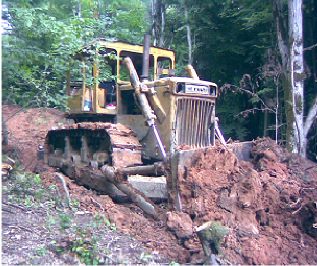
Figure 3. Excavation by bulldozer in Khul Kheil forest of Hyrcanian zone.
