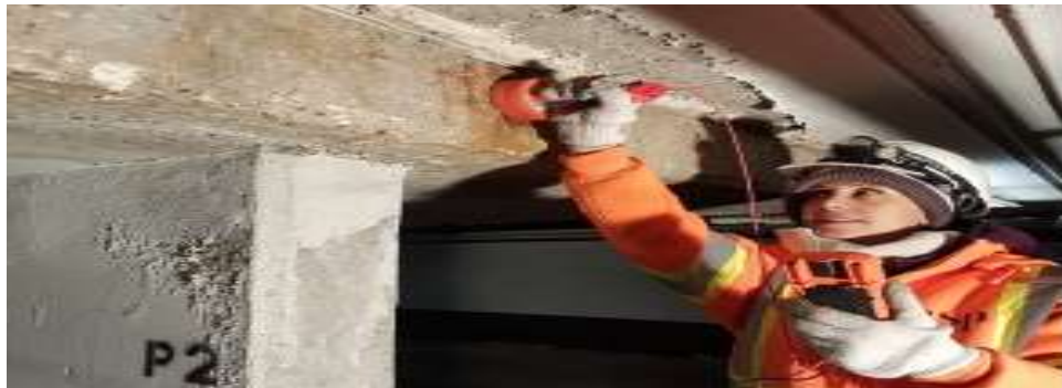
Figure 7. NDT corrosion mapping. Source: Adapted from www.fprimec.com.
