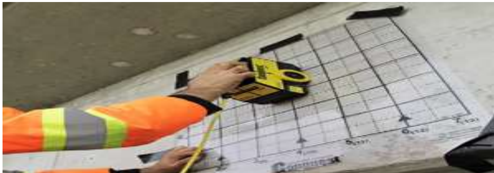
Figure 5. NDT of Concrete using GPR. Source: Adapted from www.fprimec.com.
