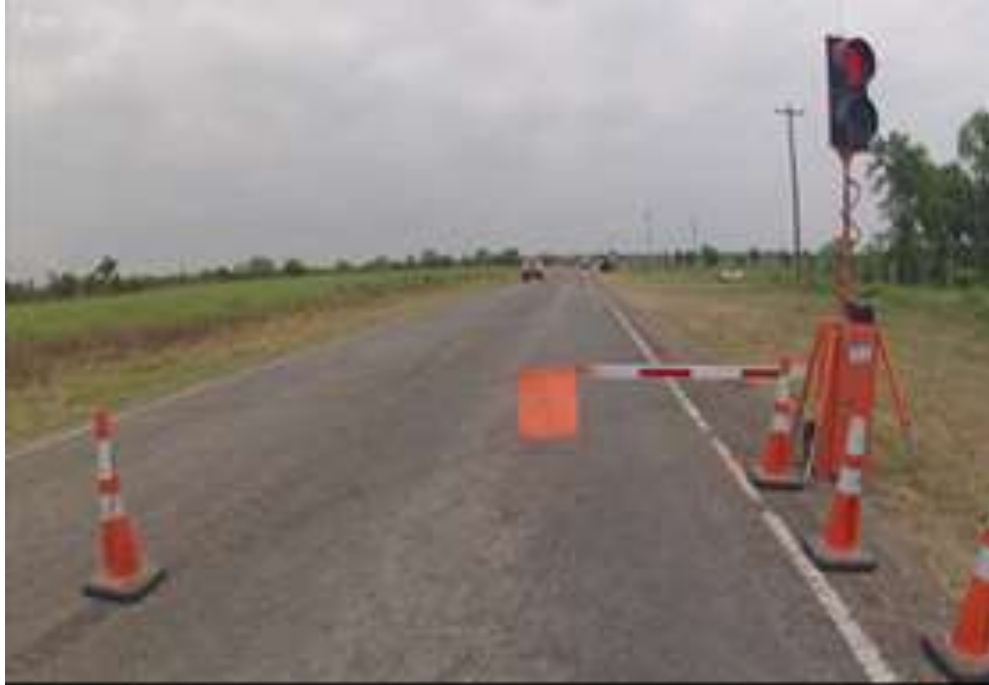
Figure 1. Automated flagging assistant device (AFAD) #1.
