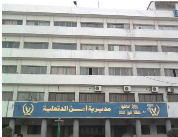
Figure 3. General view of Directorate of Security in Daqahlia Government.
